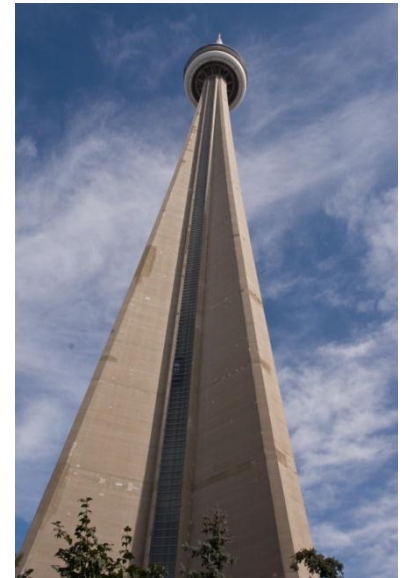
This tower uses three combiners to support 8 DTV channels, along with a single combiner for 12 FM radio stations.
